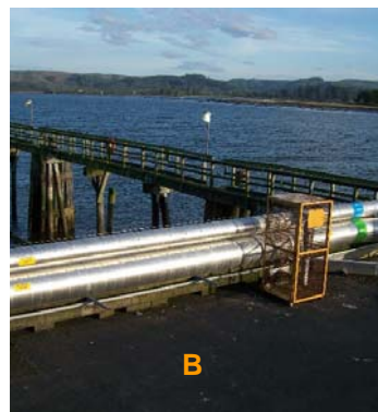
A. Port of Grays Harbor T1 is located west of the T2 Bulk Loading Facility & south of the Imperium Grays Harbor biofuels plant & site of the Westway Terminal bulk liquid facility. B. Existing creosote timber dolphins and catwalks will be removed & disposed of at an approved upland disposal site. C. T1 was built in the early 80's & longshoremen loaded barges with vanillin & lignin liquor from ITT Raynoier facilities for several years.
