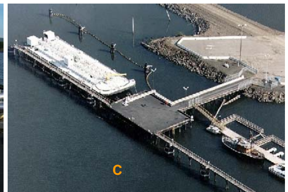
A. Port of Grays Harbor T1 is located west of the T2 Bulk Loading Facility & south of the Imperium Grays Harbor biofuels plant & site of the Westway Terminal bulk liquid facility. B. Existing creosote timber dolphins and catwalks will be removed & disposed of at an approved upland disposal site. C. T1 was built in the early 80's & longshoremen loaded barges with vanillin & lignin liquor from ITT Raynoier facilities for several years.
