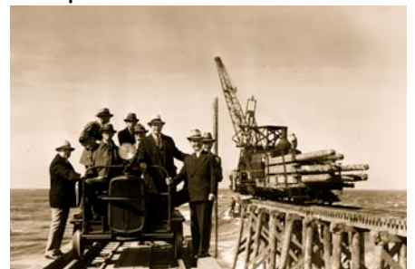
1937, officials from Washington DC and local leaders inspect the construction of the South Jetty in Westport.
