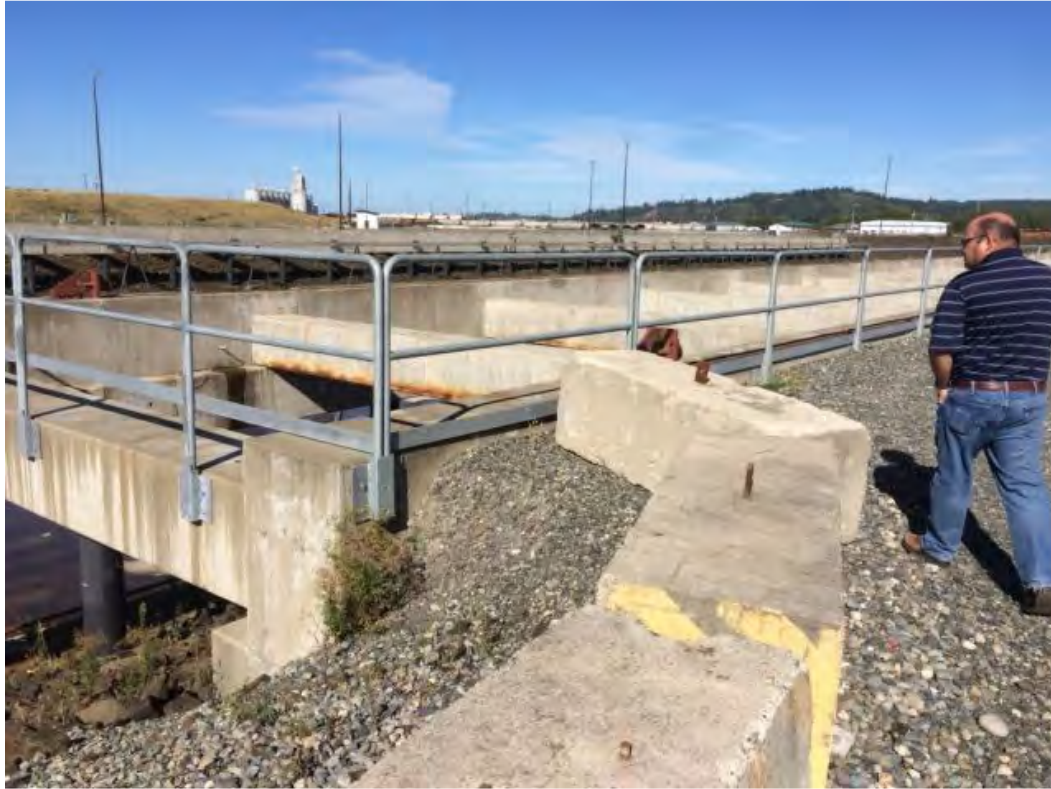
Picture 6. Crane way along east casting wall
