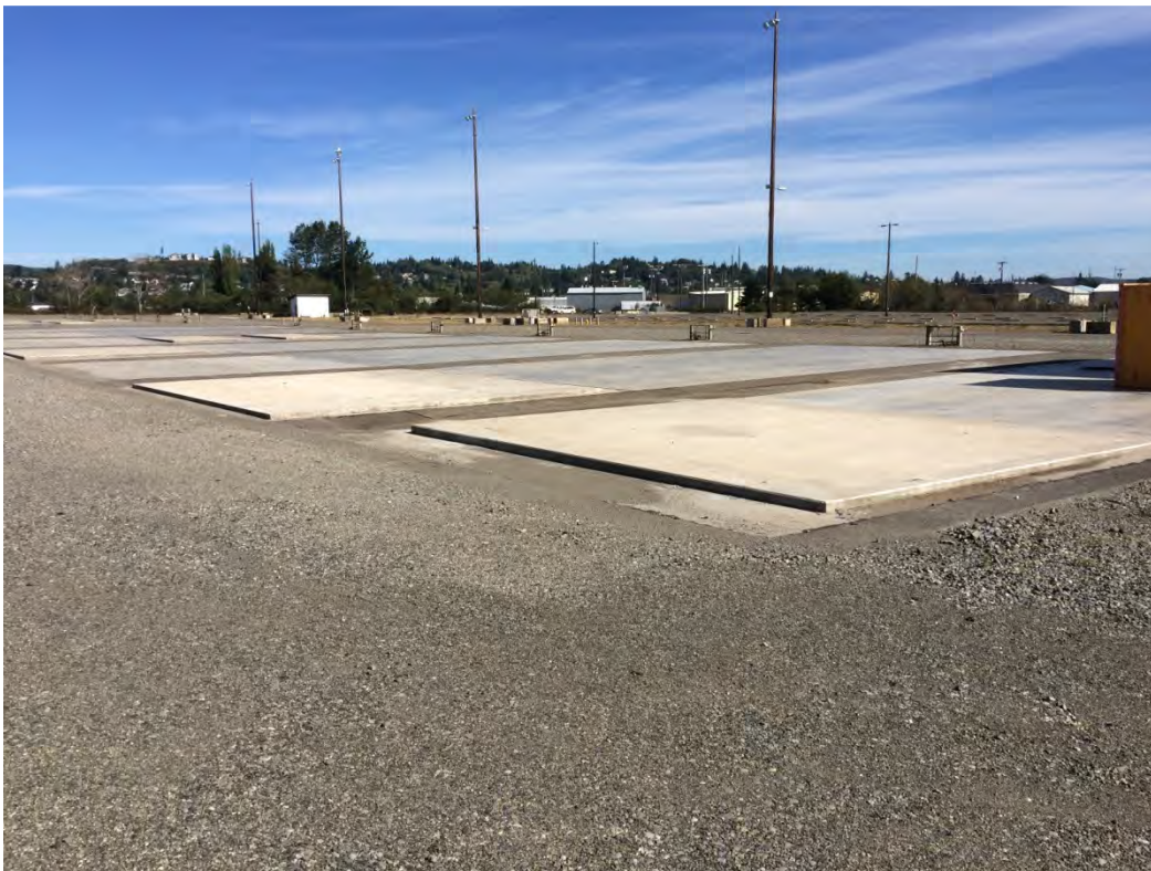
Picture 3. Raised concrete flat-panel slabs
