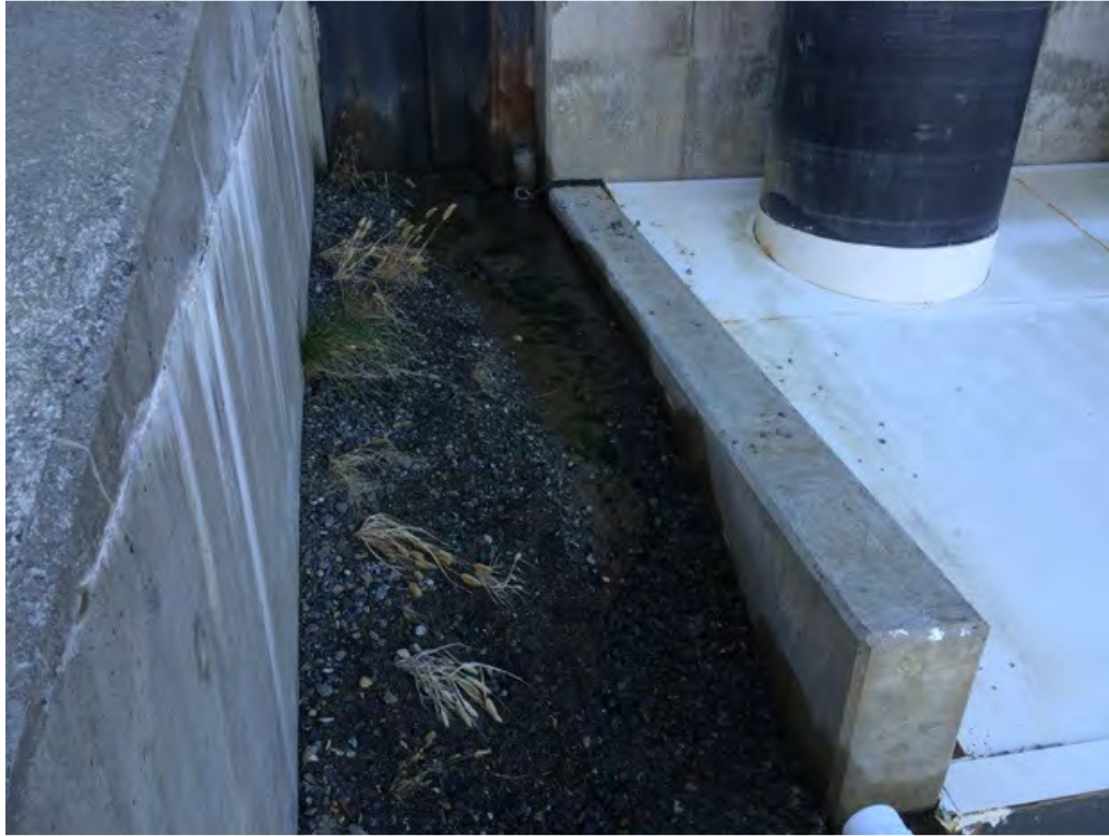
Picture 23. Leak under sheet pile wall in southeast corner of casting basin
