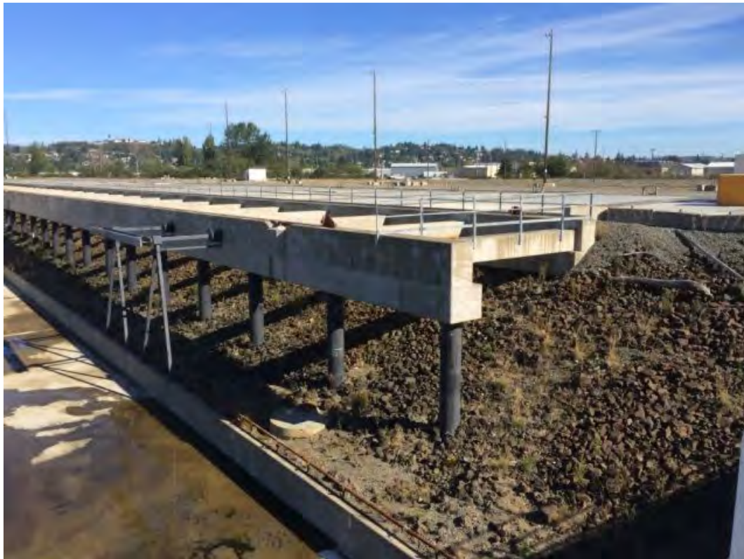
Picture 7. Crane way along east casting wall, riprap rock below
