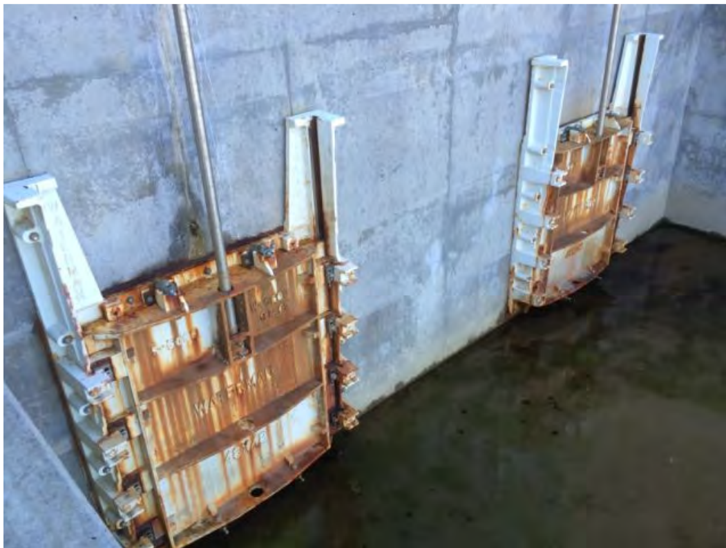
Picture 21. Remote-controlled water flooding gates in southeast corner of casting basin
